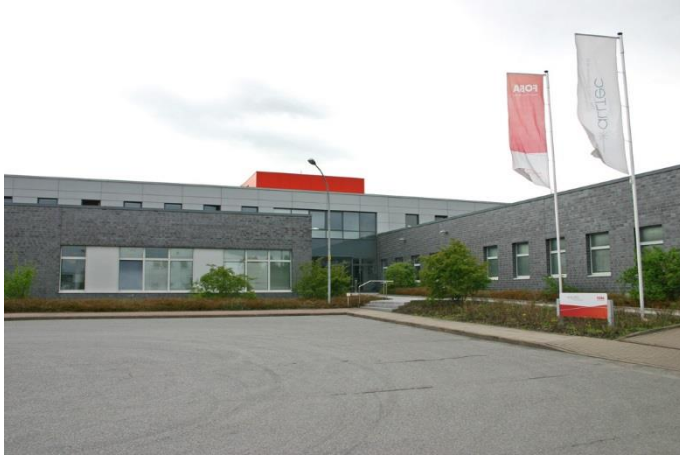
The ALLTEC facility in Selmsdorf near Lübeck. With the merger of ALLTEC and FOBA in 2009, Selmsdorf has become the sole production location. (picture rights: FOBA)
